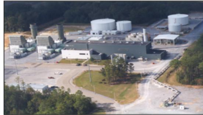
115 MW Compressed Air Energy Storage
